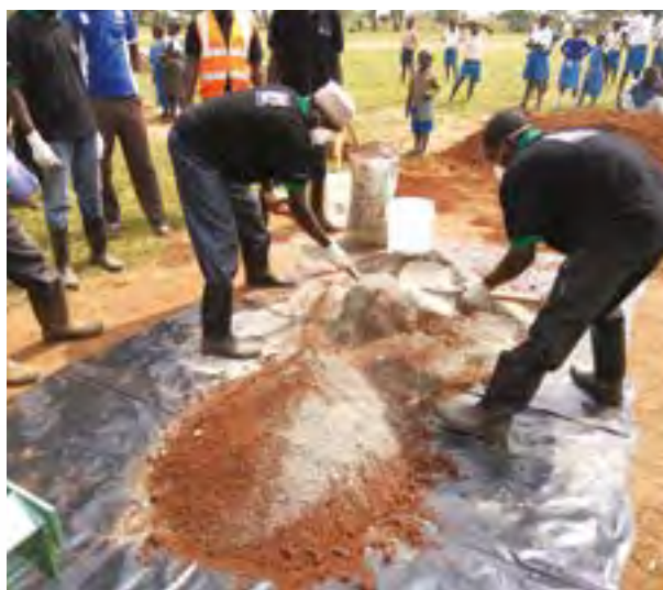
Preparing of soil Stabilised Blocks
